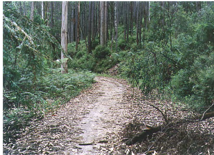
Single lane unsealed road formed but not gravelled
