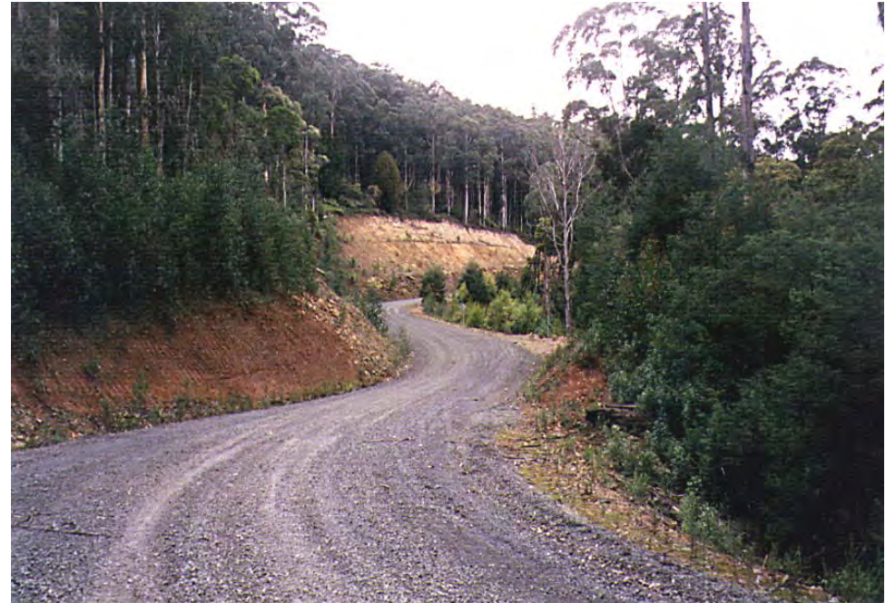
Two lane two way unsealed road
