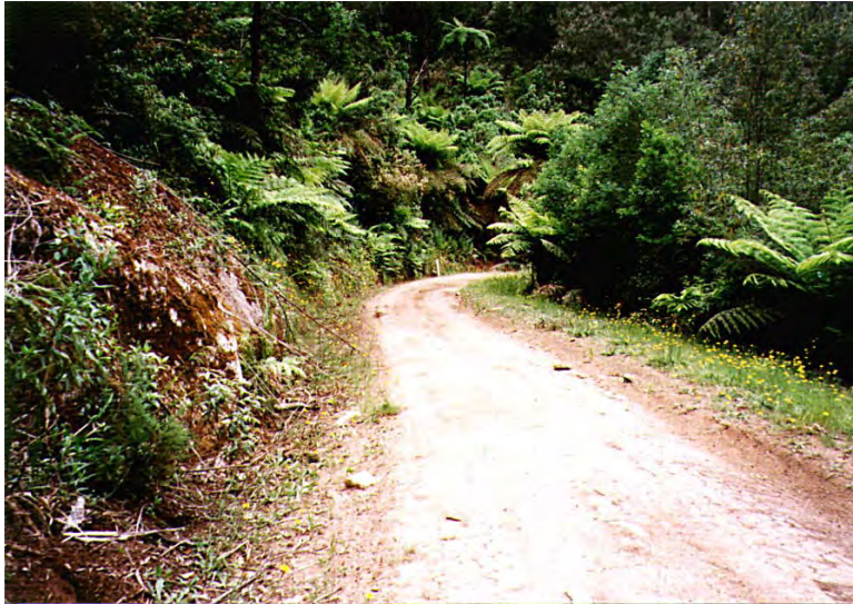
Single lane unsealed road lightly gravelled
