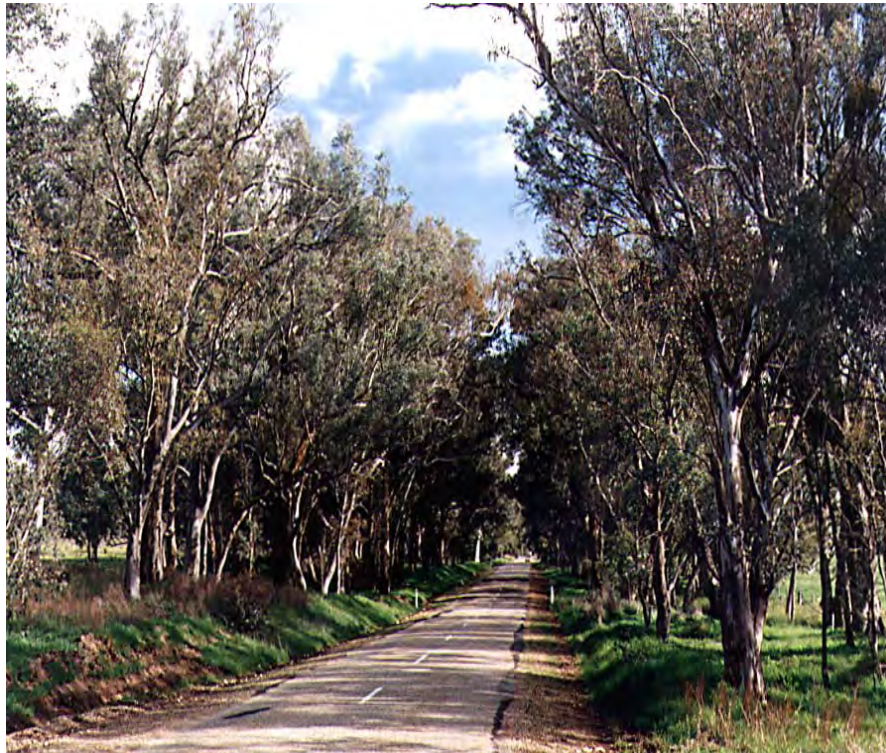
Two lane sealed road
