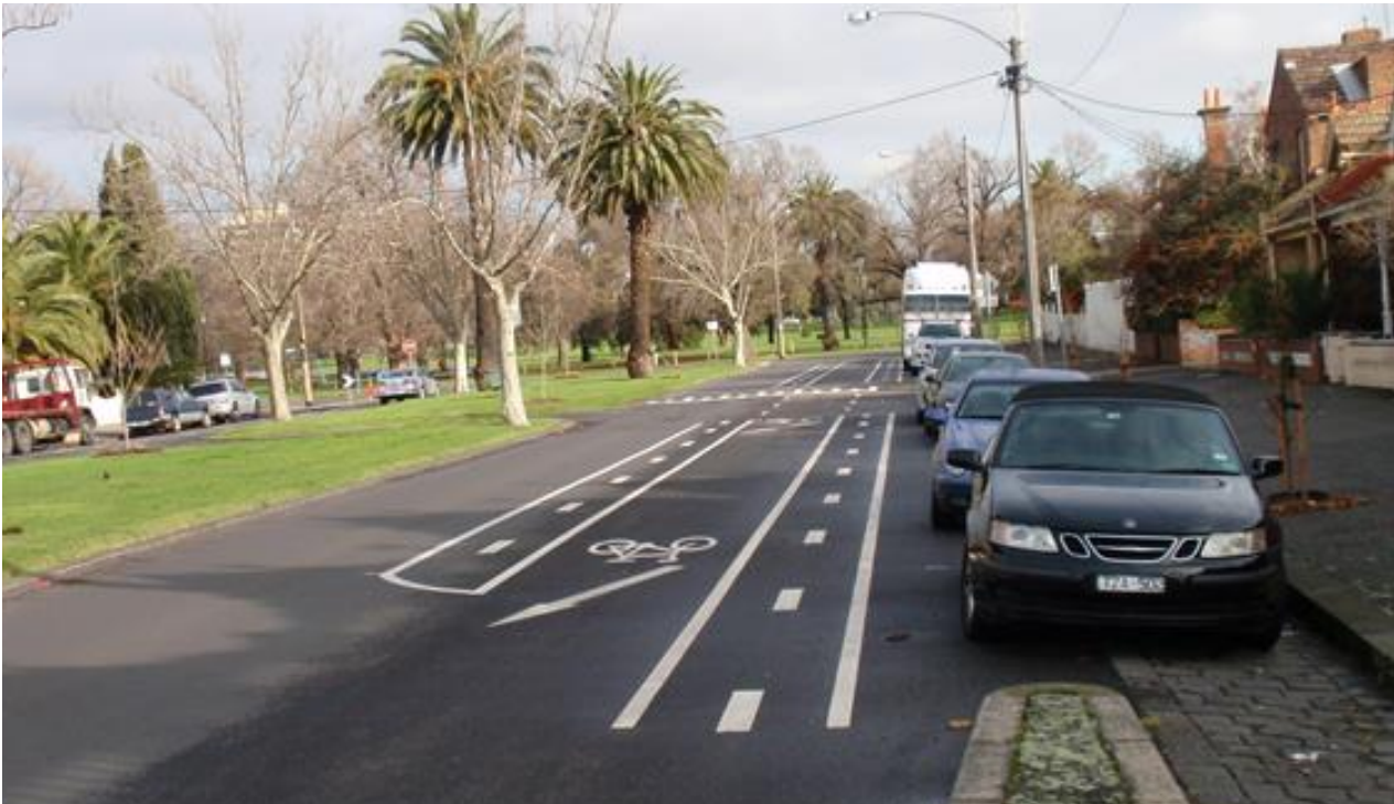
Figure 4.39: A bicycle/car parking lane with a painted separators between cyclists, parked cars and the traffic lane
