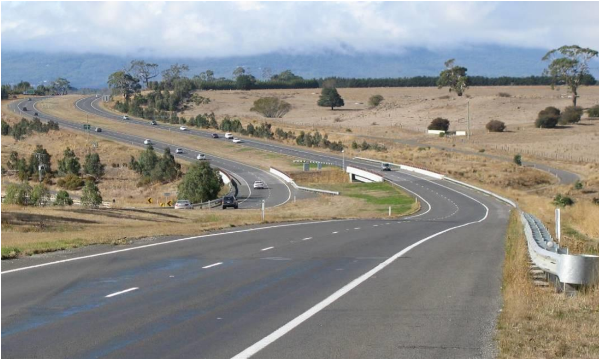
Figure 6.12: A road that is not well fitted to the terrain
