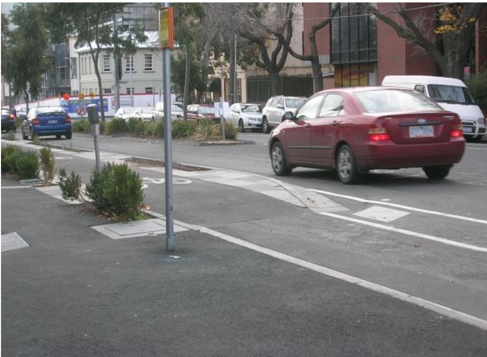
Figure 4.31: Kerb separated bicycle lane
