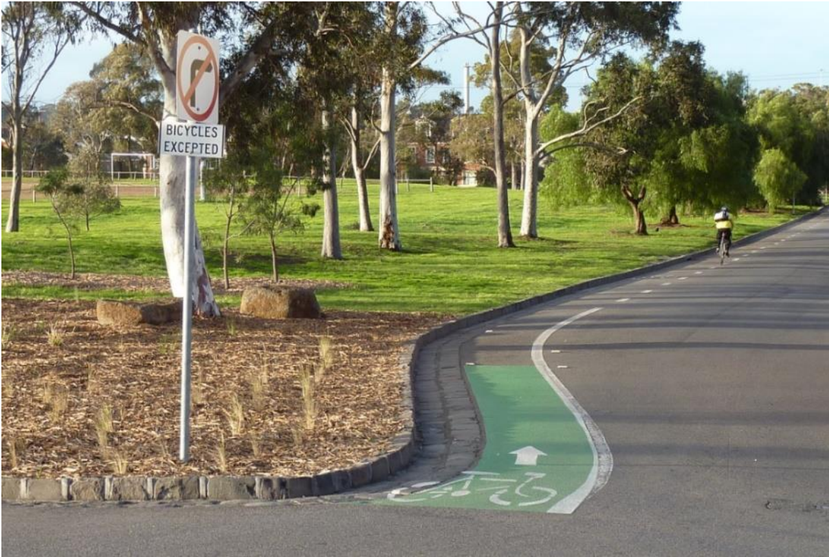
Figure 4.34: Contra-flow bicycle lane – layout
