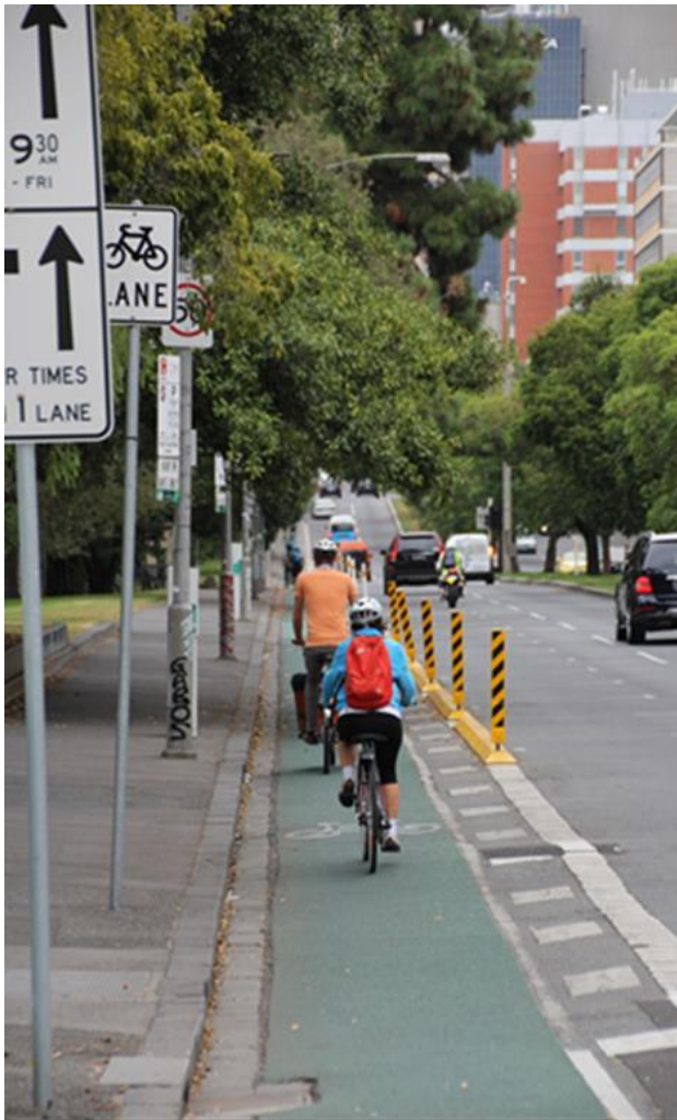
Showing peak flow direction with parking prohibited
