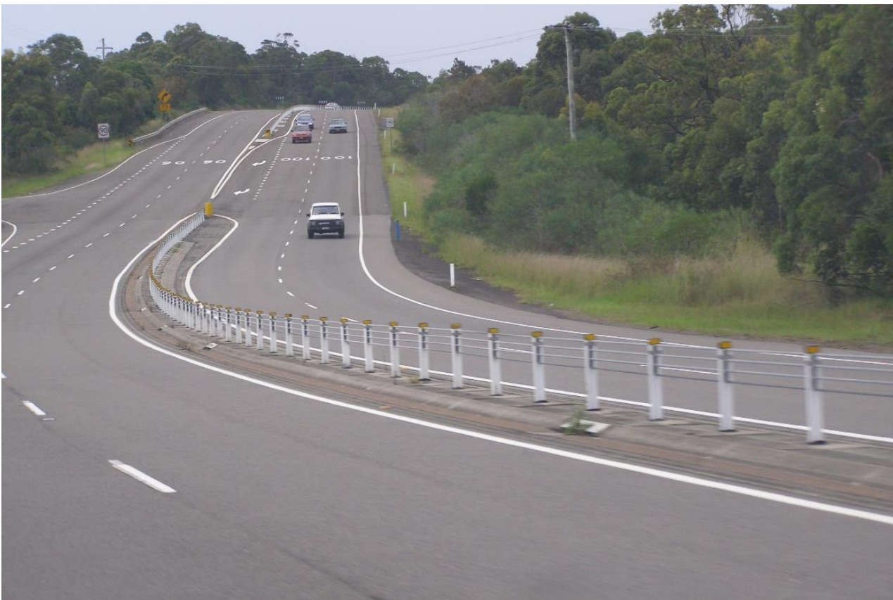
Figure E 1: Narrow median with flexible barrier (i.e. wire rope safety barrier)
