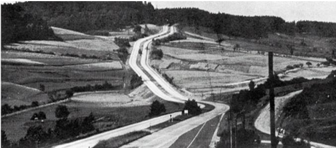
Figure 6.12: A road that is not well fitted to the terrain
